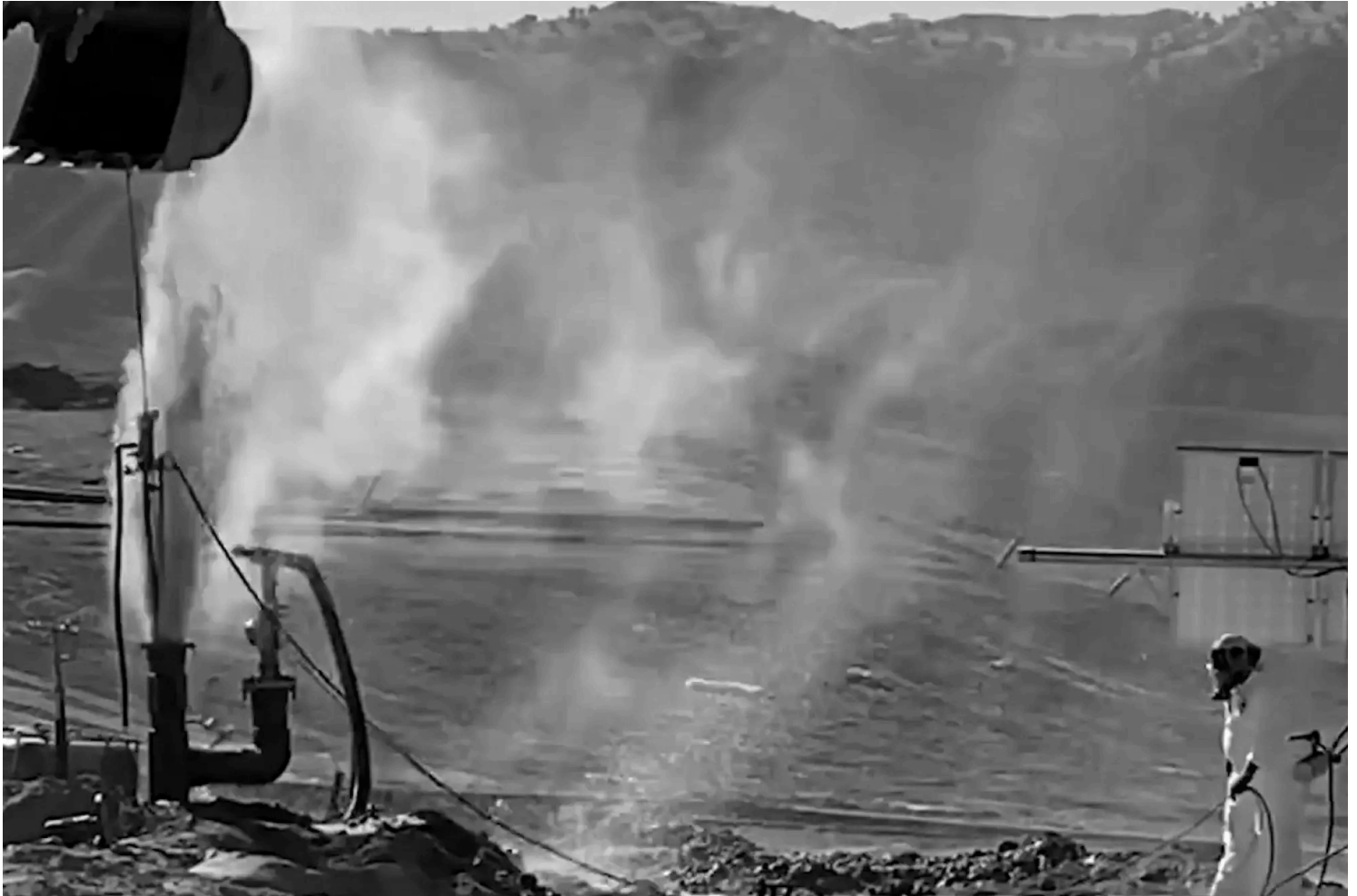
Contaminated liquids erupt onto the surface of Chiquita Canyon Landfill in Castaic in November 2023. (South Coast Air Quality Management District)
