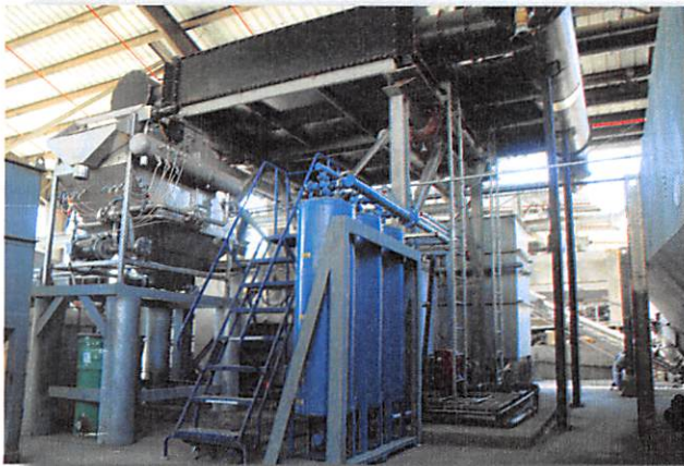
Biosolids Drying Facility
